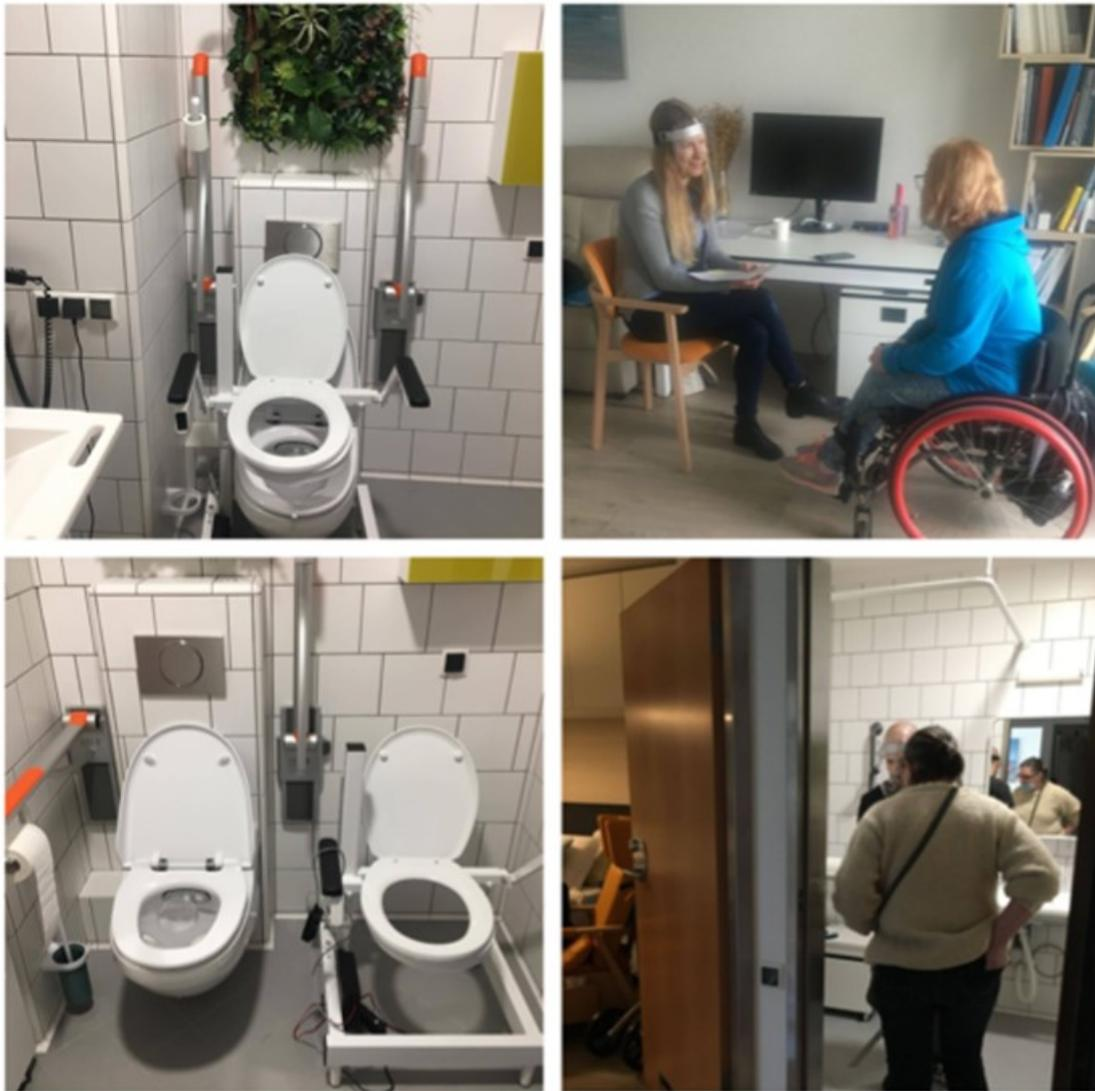
*Figure 3: The testing in Poland. GEBERIT AquaClean 8000 with an additional PW GAMA lift next to it (top left) and installed on the existing toilet (bottom left). Participants of the testing - a primary user during the interview with the OSF team member (top right) and caregiver visiting the restroom (bottom right).*
